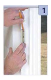
Place latch in door jamb against inside edge. Holding latch firmly, mark holes. Drill 1/8" pilot holes. Install latch using enclosed screws.
